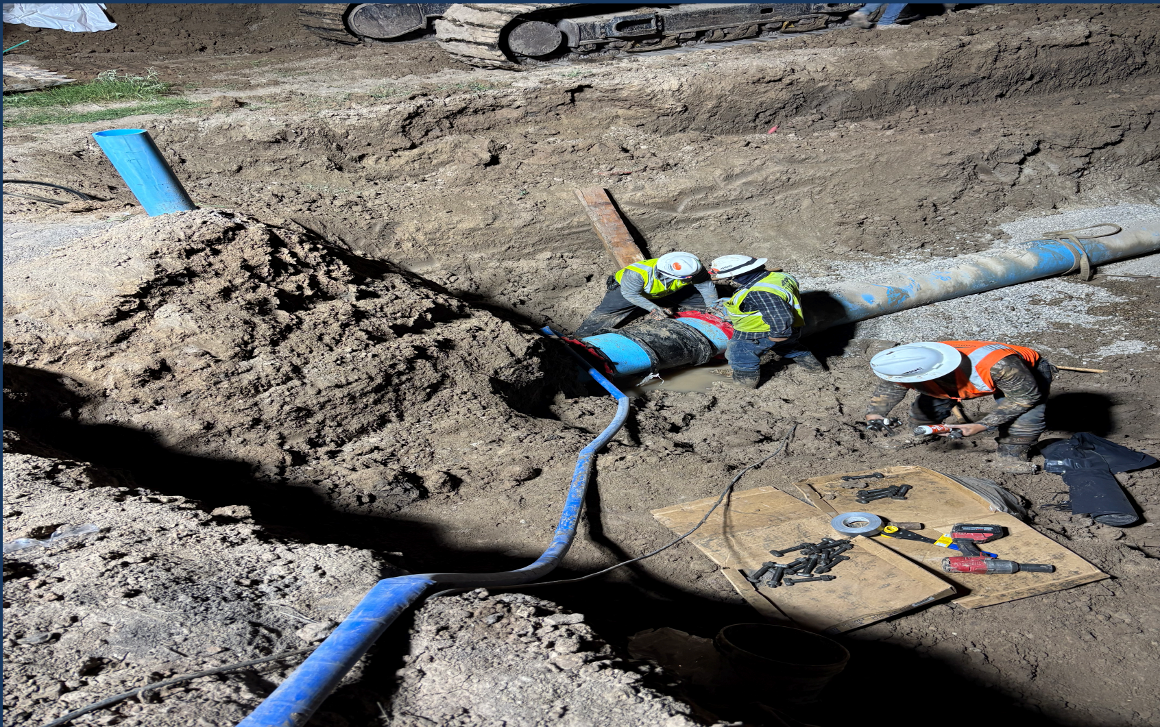
S. CAGE 18" WATER LINE RELOCATION STA. 1087+93
